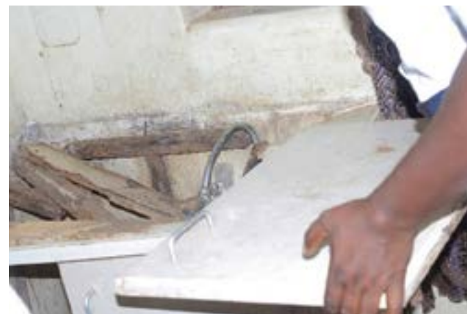
HDU sink before expansion and remodeling
